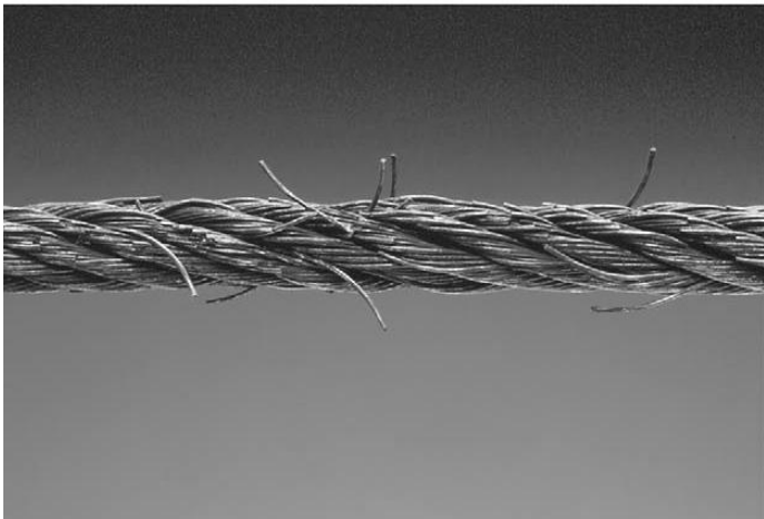
Cable With Severe Corrosion
